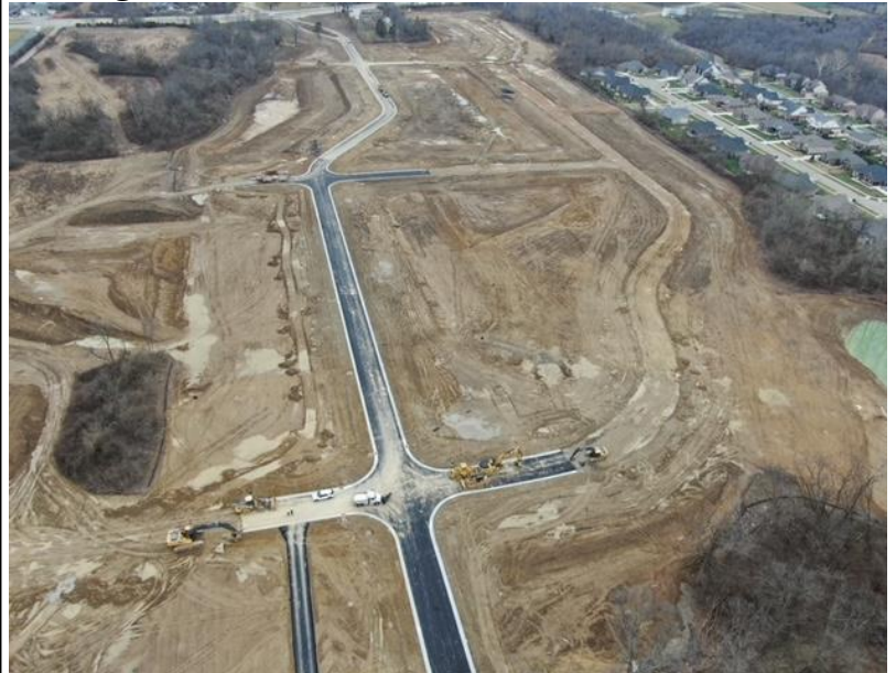
Looking South towards Rt. 4
